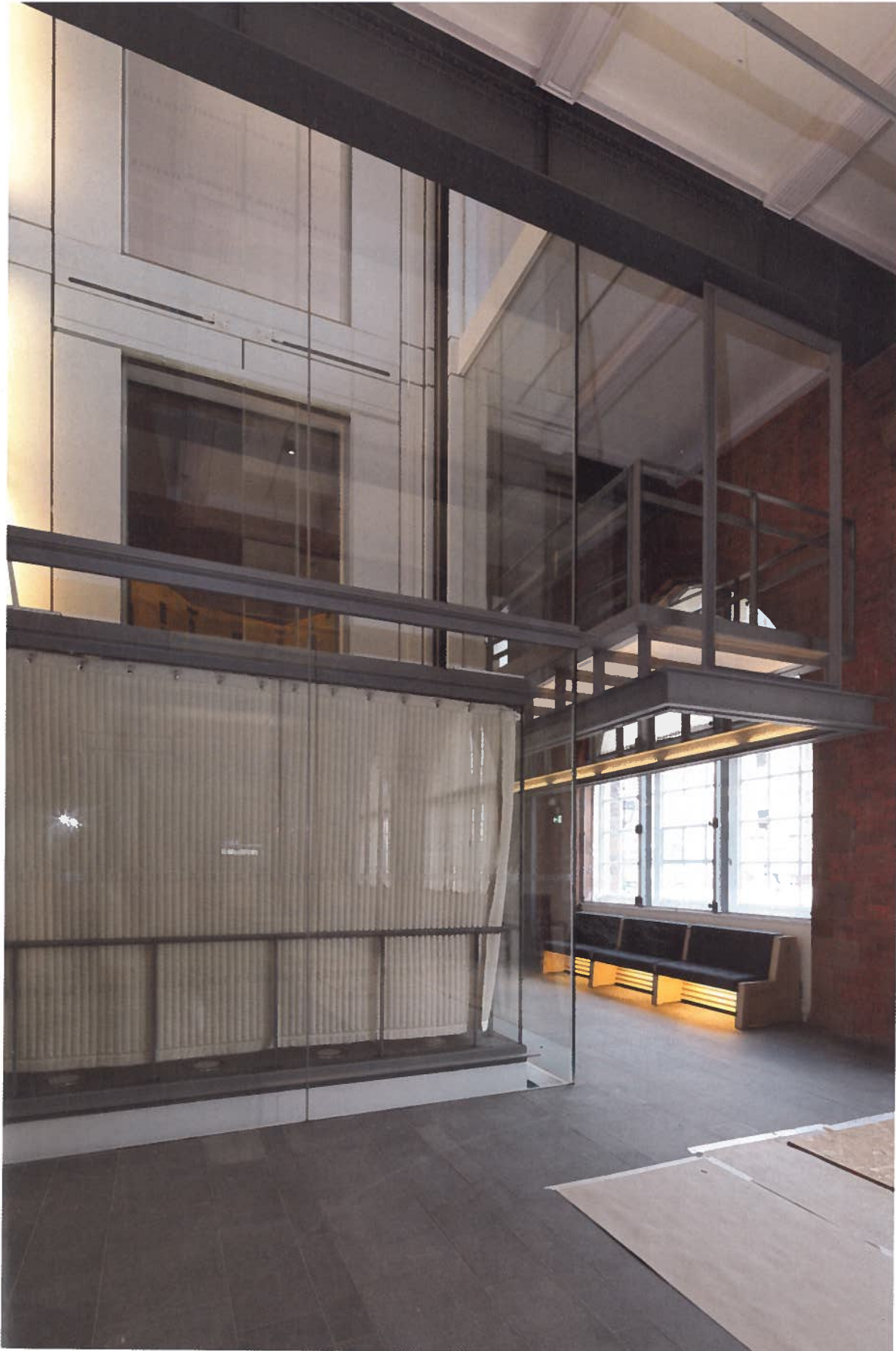
A 48-person capacity lift made entirely of glass runs through the core of the building
