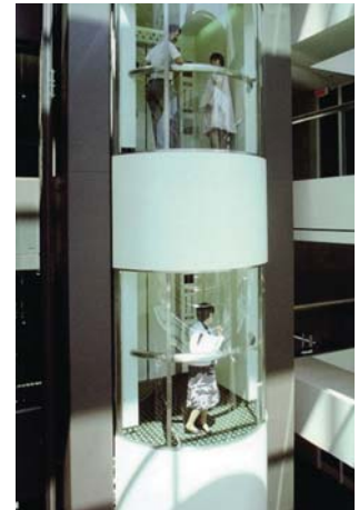
Designers for the Broadgate Tower (above) and The Shard (below) have incorporated double-deck lift technology
